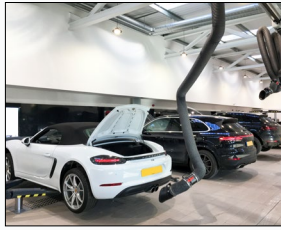
Exhaust Extraction Systems.
